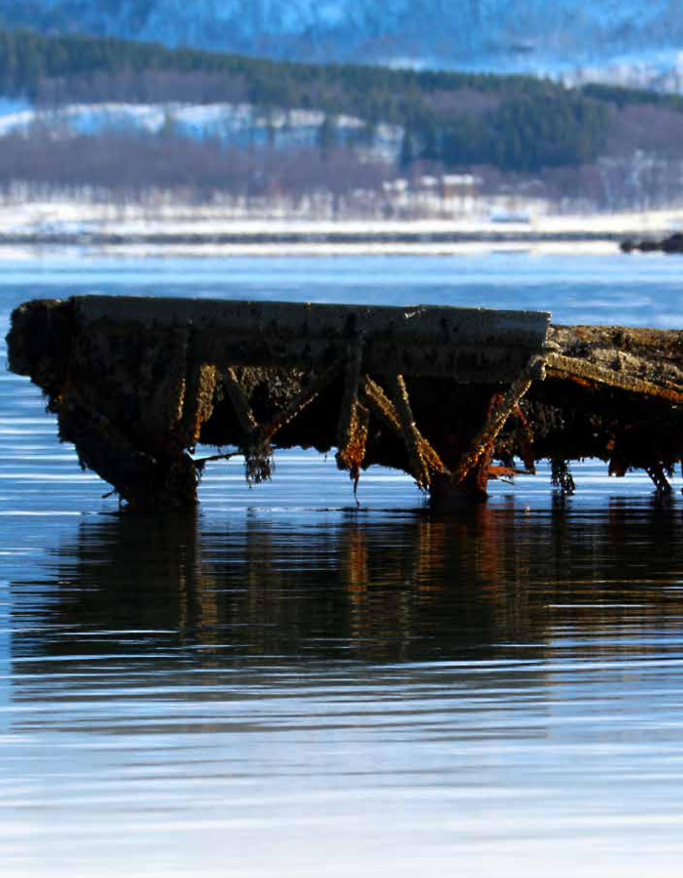
Tirpitz salvage wharf structure, 2023.
